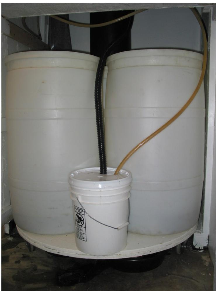
*Figure 1.1: Completed composter. Hose from urine-separating seat to bucket in front.*
